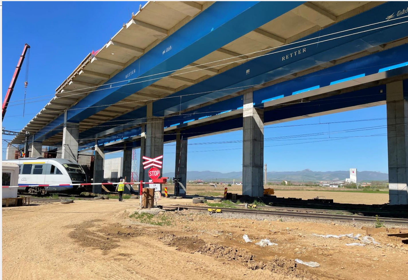
2021 Motorway overpass on Sebeș -Turda, L = 217\text{m}
